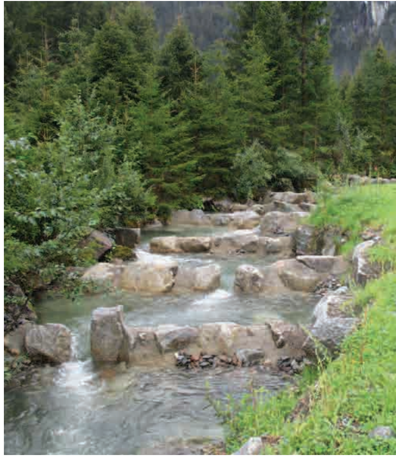
The new pool and weir fish ladder
