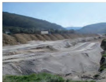
Dumping of the dike on the right side
