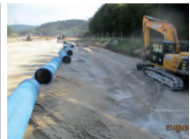
Laying of water pipe DN500
