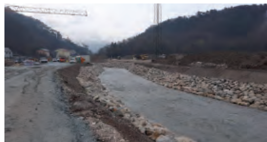
Diversion channel for the Triesting
