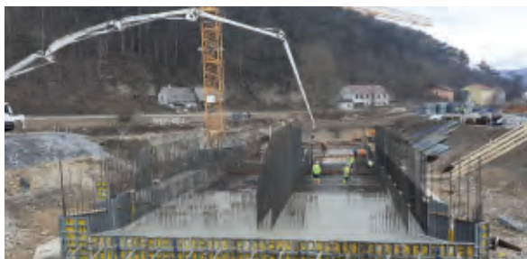
Construction of the base plate of the bottom outlet construction
